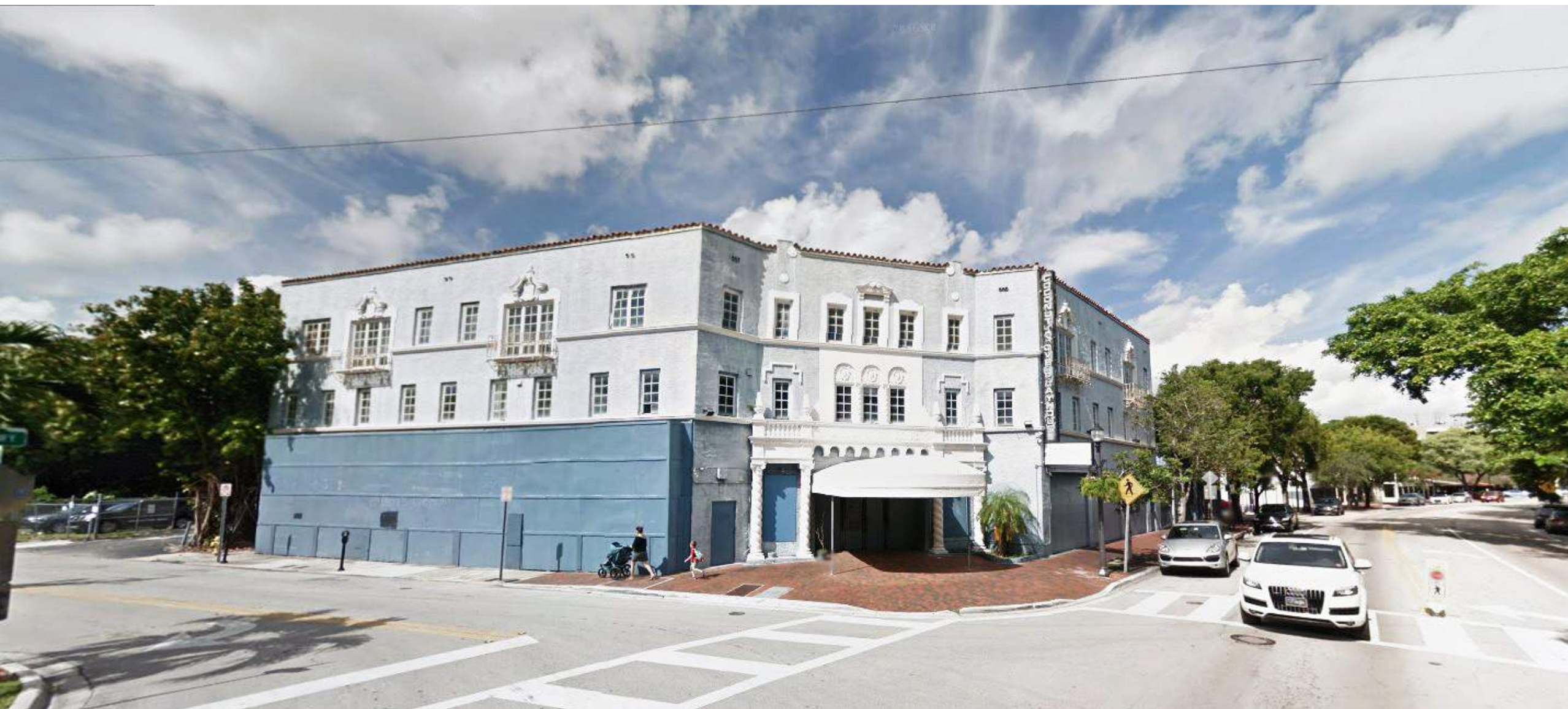
EXISTING SITE CONDITION
