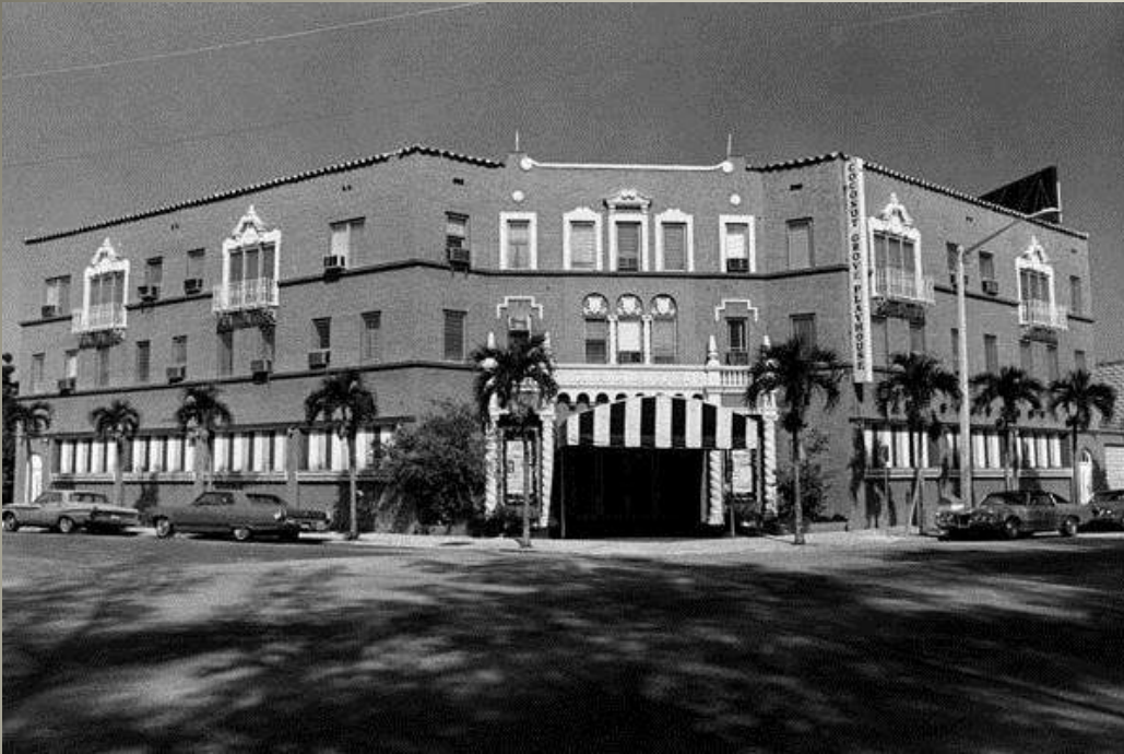
Coconut Grove Playhouse front elevation showing the closed up store fronts (Photo 1971)
