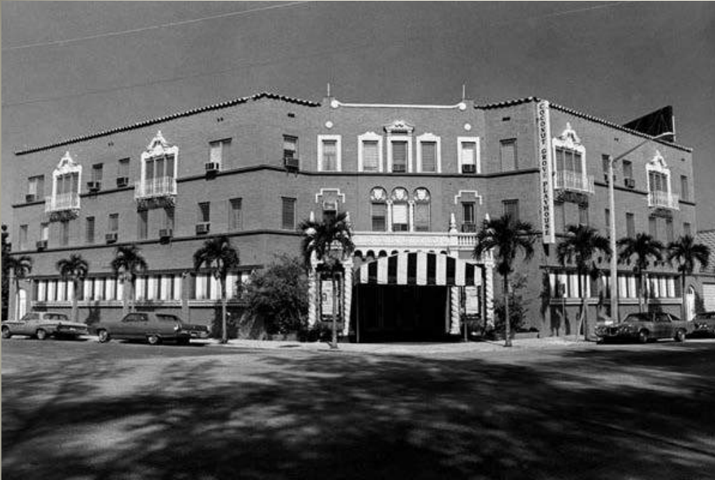
Coconut Grove Playhouse front elevation showing the closed up store fronts (Photo 1971)
