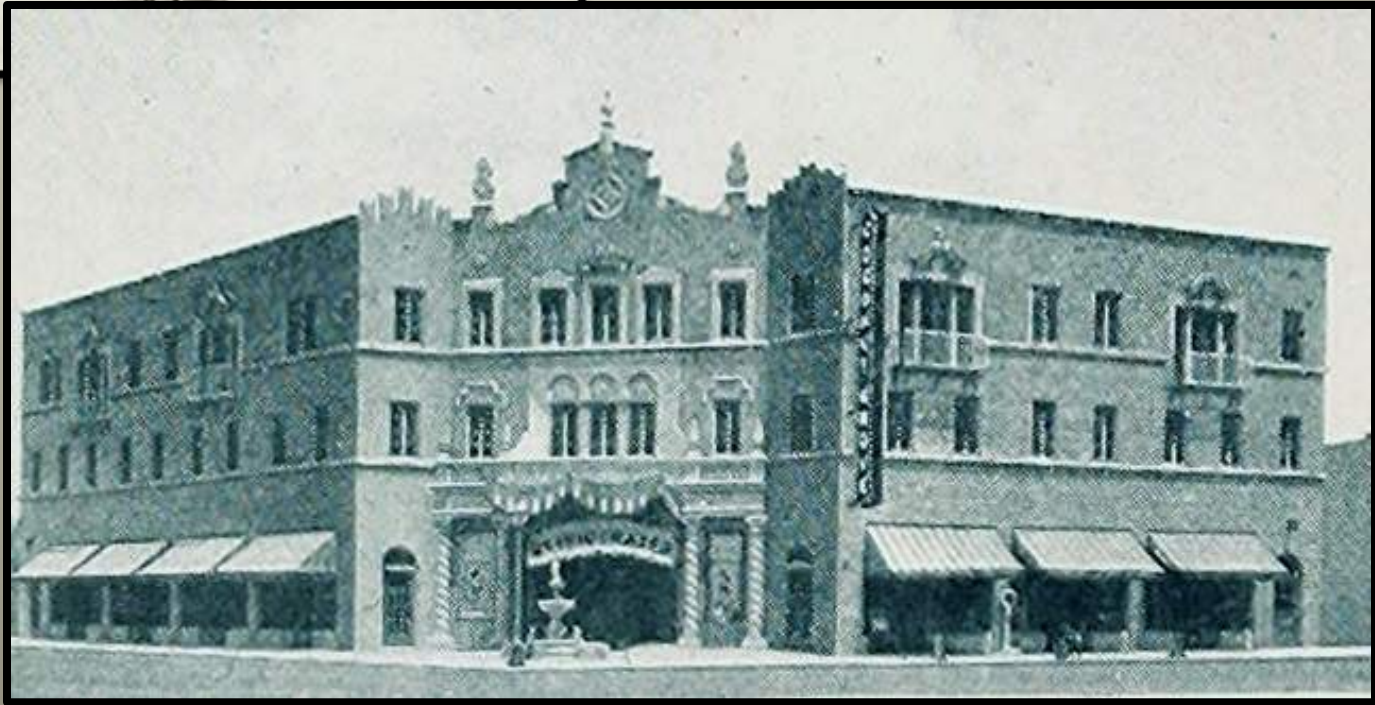
Exterior view of the Paramount Theater in Palm Beach and the Coconut Grove Playhouse
